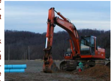
Construction on the Markland Business Park began in November.
